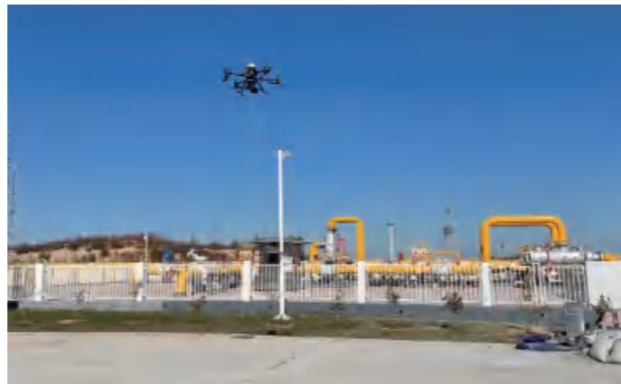
Drone Leak Detection
