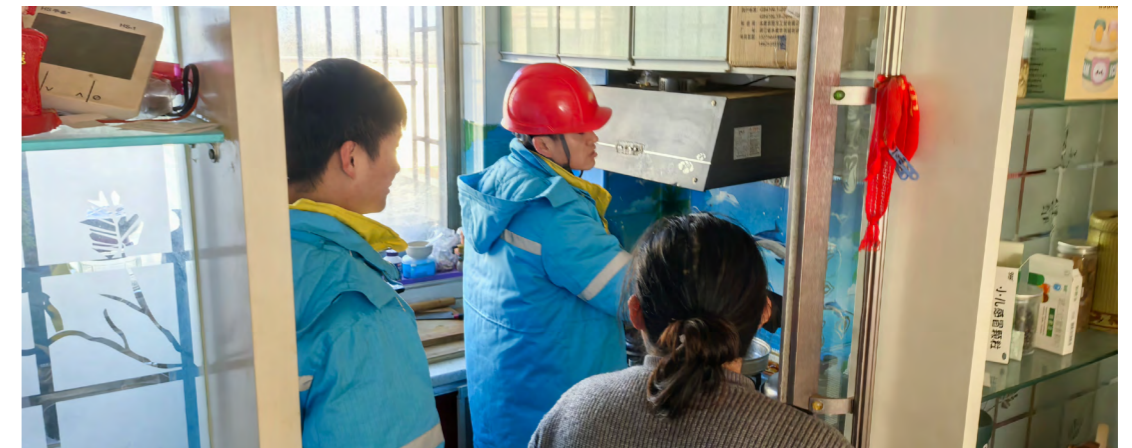
“煤改气”通气点火现场
