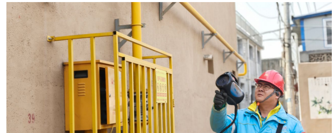
Rural Gas Pipeline Infrastructure Safety Inspection Checks
