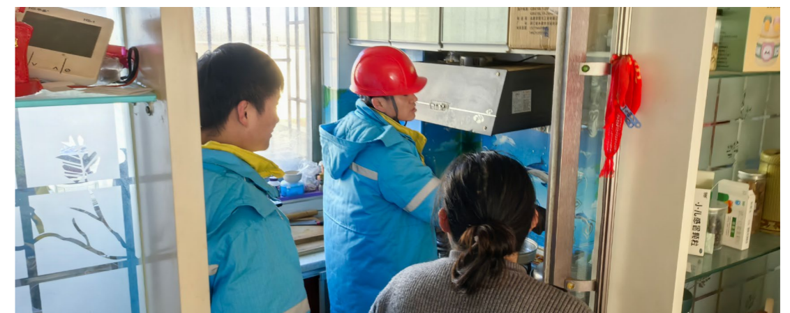
"Coal-to-Gas" System Ignition Scene
