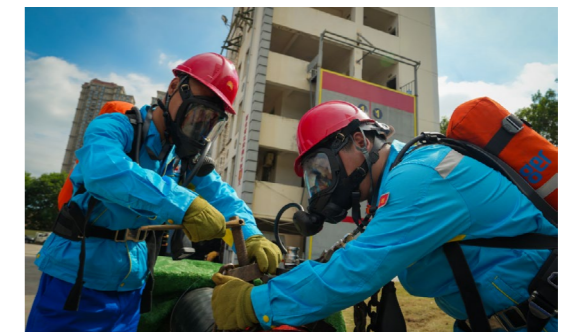
Steel Pipe Plugging
