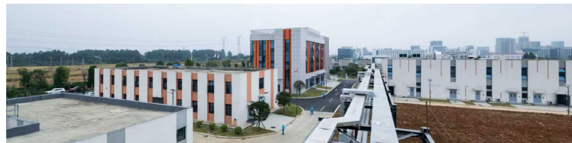
Energy Station Facility Area
